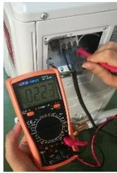
2) If the 1 & N which connect to indoor unit voltage is normal, measure the voltage between the outdoor terminal 1 and N. If the voltage change occurs between 0~24V (change pulse voltage), please replace indoor main PCB.
