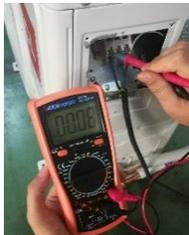
3) If the 1 & N which connect to indoor unit voltage is normal, measure the voltage between the outdoor terminal 1 and N. If the voltage change occurs between 0~12V( change pulse voltage), but there is no 24V, please replace the outdoor PCB.
